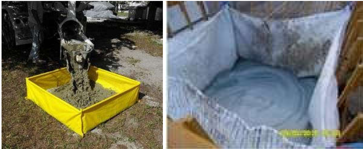
Plate 10.1 and Plate 10.2: Example Photos of Concrete Washout on Site Fuels and Chemicals
